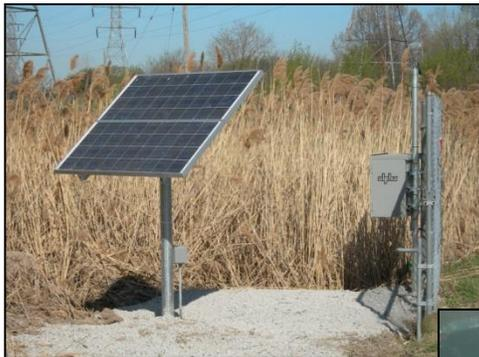
Greenstar was able to install a 4.5' x 4.5' solar panel instead of the 9' x 10' that would have been required for 24/7 winter use.
